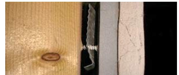
Incorrect screw size breaching the flexibility of the resilient bar and hence compromising the performance of this partition.
