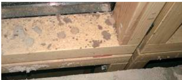
The sealing between different constructions needs to be considered carefully. Image of junction between mullion and floor slab.
