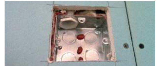
Acoustic putty poorly installed, still a large gap around the electrical socket.
