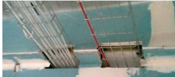
Cable tray passing through separating walls. This is impossible to acoustically seal.
