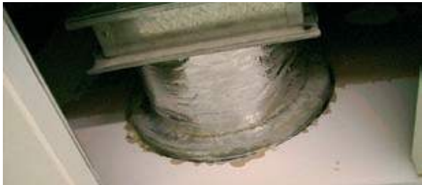
No patressing around cross talk attenuator, the cross talk should also straddle the partition, rather than installed on one side only.
