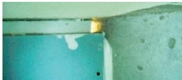
Gaps principally at the head and facade of partition interface. A major reason for on site shortfalls in sound insulation levels.
