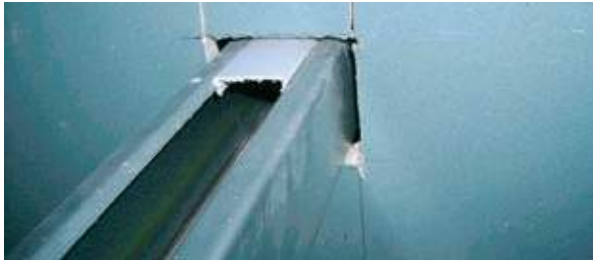
Electrical trunking not packed with sand bags, large gaps around the penetration point, no patressing
