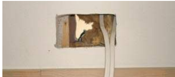
Back to back electrical sockets breaching the performance of the separating wall.
