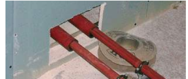
Pipe work hidden by raised floor, no patressing or sealing of any sort. Fails to meet acoustic requirements.
